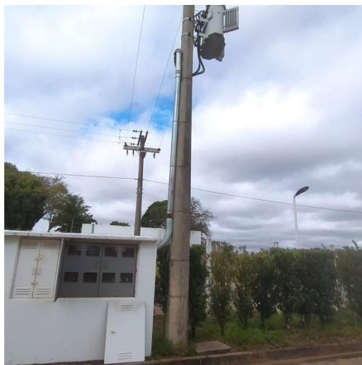
Vista geral – Quadro Principal
