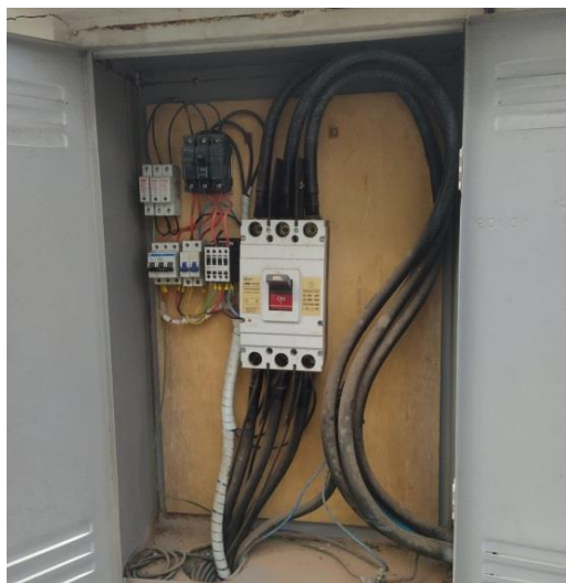
Disjuntor Geral Principal – 300A
